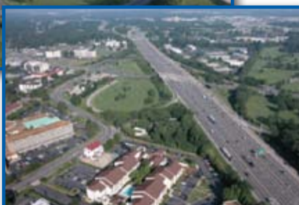
Aerial view of Newtown Interchange, looking west
