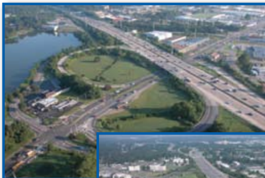
Aerial view of Witchduck Interchange, looking west
